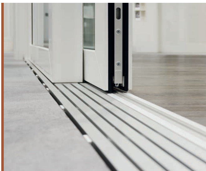
Lift&Slide element (PVC) with GU-thermostep, barrier-free
